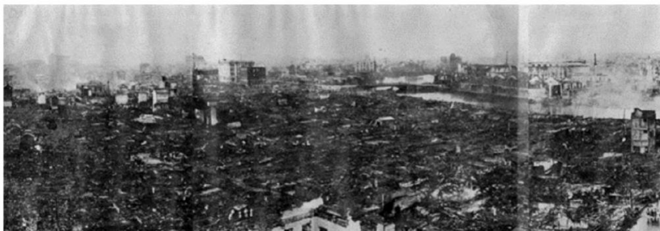
Desolation of Nihinbashi and Kanda as seen from the roof of the Dai-ichi Sogo Building
